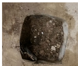
Shower drain repairs underway
